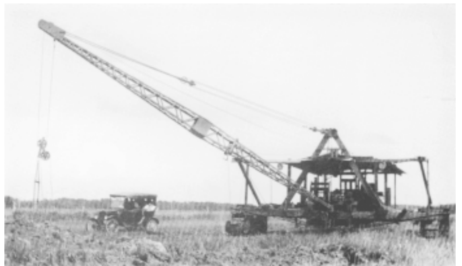
Road building in the Steinbach area in the 1920s. This dredge was owned by "Fast Brothers" of Kleefeld--Henry D. Fast, George S. Fast and Neil S. Fast. Drainage was a perennial problem throughout the Hanover Steinbach area until the construction of the Manning Canal in 1908 and the Tourond drain, cutting across Hanover from the Sarto corner on P.T.H.12 to Kleefeld and west to Otterburne. Photo courtesy of Is there any place like it? page 22.
