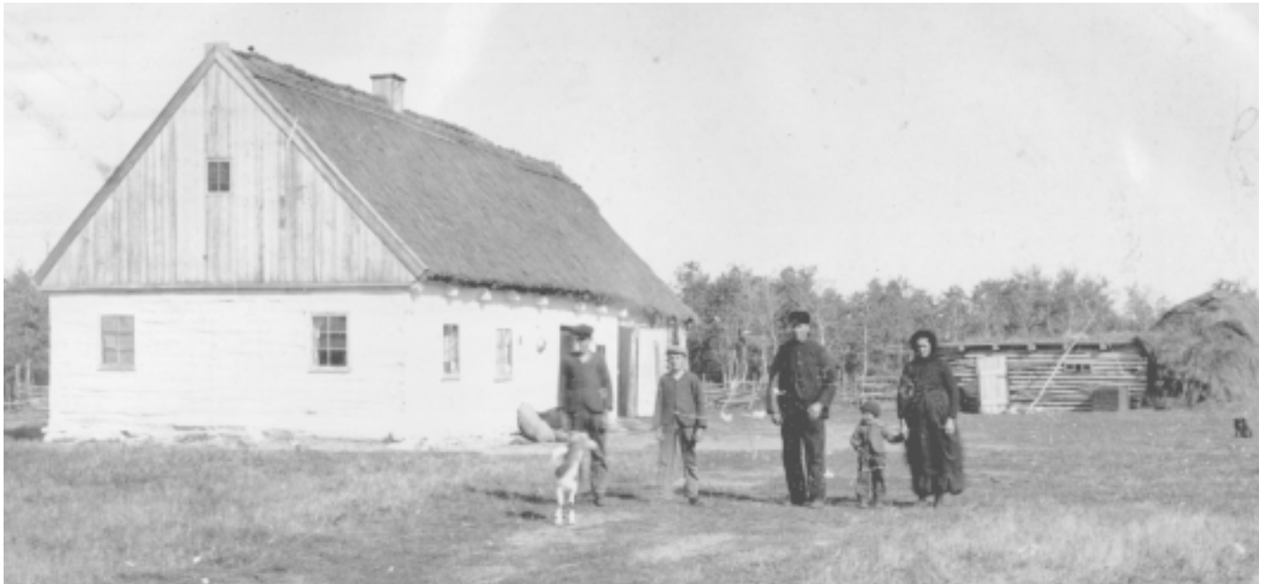
The log house was an intermediate stage between the hastily constructed sod huts and log shanties and the traditional wood-framed housebarns. Although this house-barn was only built circa 1884 it is representative of this type of construction on the East Reserve. It was built by Jakob Dueck, Rosengart. Standing in front of the building are, l. to r.: Jacob N. Dueck, Diedrich N. Dueck, Jakob Dueck (b. 1846), grandson Jacob Ginter (son of Jacob Ginter and Anna Dueck), and Maria (Neufeldt) Dueck (b. 1846). This house still stands on SW18-6-6E. Photo taken facing northwest, circa 1895. Courtesy of Mrs. Elizabeth Friesen/Linda Buhler.
