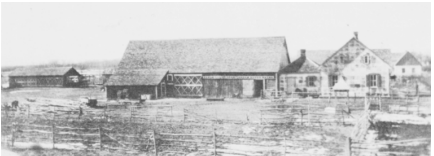
A housebarn in Alt-Bergfeld built in 1904. The prosperous Wirtschaft belonged to the Peter T. Falk family. This structure already shows some innovation and adaptation to North American conveniences and construction methods. The housebarn was no longer under one roof line and actually consisted of separate house and barn joined in the middle by the milk house and/or summer kitchen. This had become a common style of construction on the East Reserve by the 1890s. Photo courtesy of Grunthal History, page 55.
