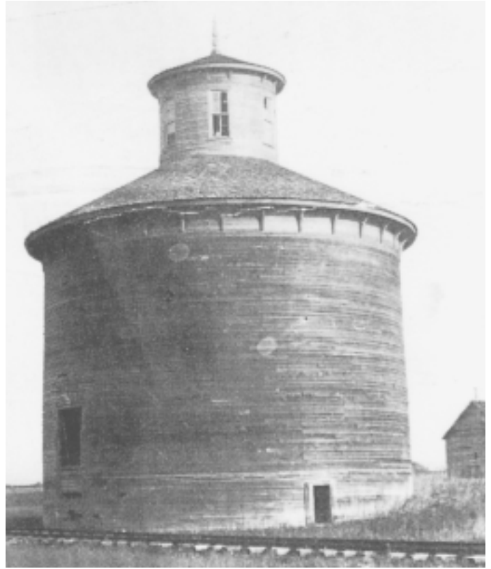
Western Canada's first grain elevator built in Niverville in 1879 by William Hespeler. The structure was constructed of timbers brought by river boat from Moorhead, Minnesota. The 25,000 bushel elevator was situated a few hundred feet from Kaiser Street, now Main Street. The elevator served Niverville for 40 years. Photo courtesy of Reflections, page 351.
