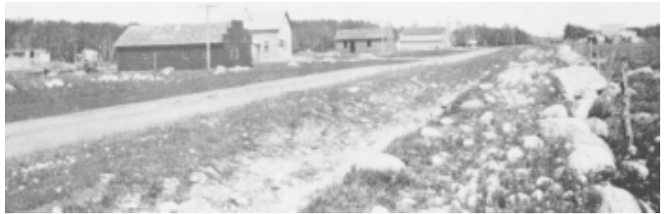
The “new” Grunthal Main Street, 1937. Photo courtesy of Grunthal History, page 113.
