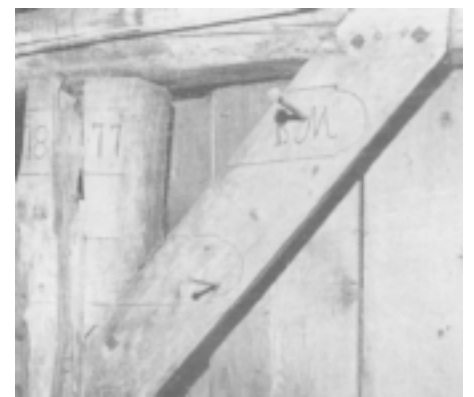
The Mennonite pioneers built their buildings to last. It was customary on completion of the building in the building supervisor to carve his initials and date of completion onto one of the upright beams. The initials on the Jakob Wieler housebarn in Eigenhof read "B.M." and the date is "1877". The photograph shows the huge axe-hewn beams and wooden pegs typically used in early construction. Photo courtesy of Reflections, page 32.
