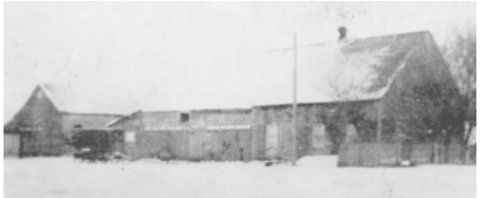
Jakob L. Plett house barn on NE25-7-6E built in the old Blumenhof village and moved onto his homestead in 1890. The building plan followed the traditional pattern and utilized homemade cedar shakes as sheathing material. The hay shed at the rear is reminiscent of the “Quere Scheune” hay shed built diagonally across the rear of many larger Wirtschaften in Russia. Photo courtesy of Plett Picture Book, page 134.
