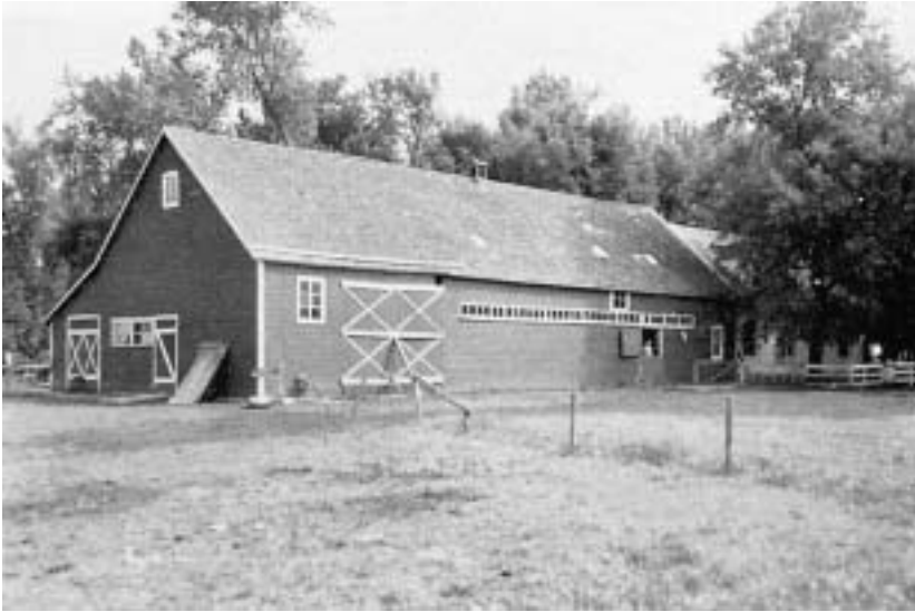
TYPICAL MENNONITE FARM BARN AND HOUSE AS SEEN FROM THE BARNYARD
