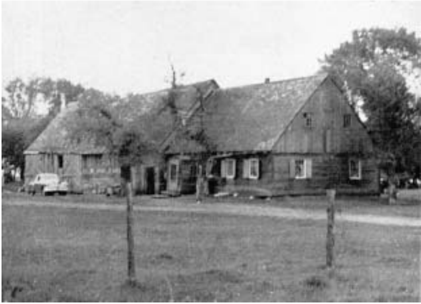
AN OLD FARM HOUSE IN NEUHORST (WEST RESERVE)
