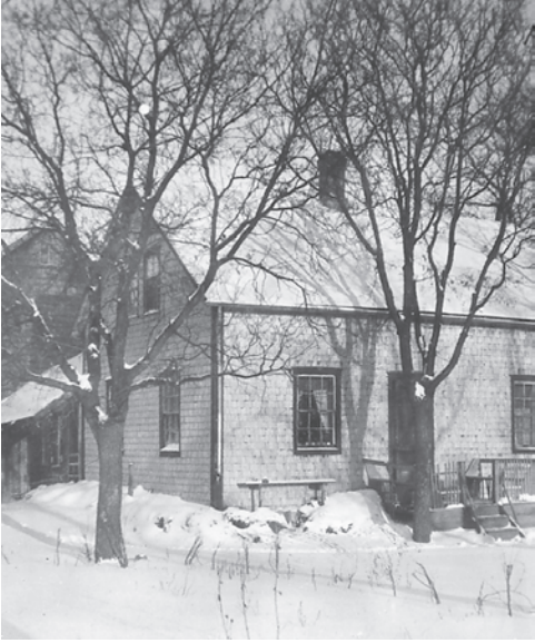
A photograph of the Johann R. Dueck house-barn located directly across Main Street from the E.M.C. (formerly Kleine Gemeinde) church in Steinbach. The structure was built in a "L" shape, with a summer kitchen between residence and the barn. The property was acquired in 1928 by Mrs. Susanna Siemens Neufeld, who took this picture on December 8, 1935. 869 Photo - Preservings, No. 10, Part One, page 74.
