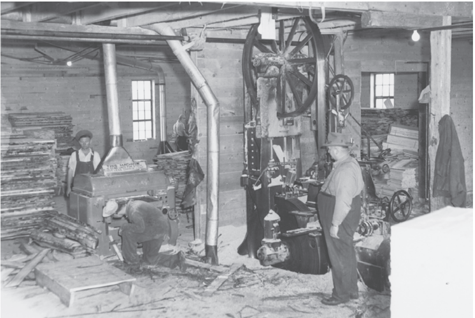
Co-owner, Jakob R. Plett, showing the interior of the box factory, 1953. Photo - Eugene Derksen.
