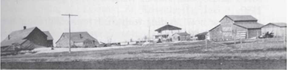
Early farmyard built up by Peter K. Goossen in Rosenort, Manitoba. The large house and farm buildings testify to a prosperous farm. Photo - Furrows in the Valley, page 417.
