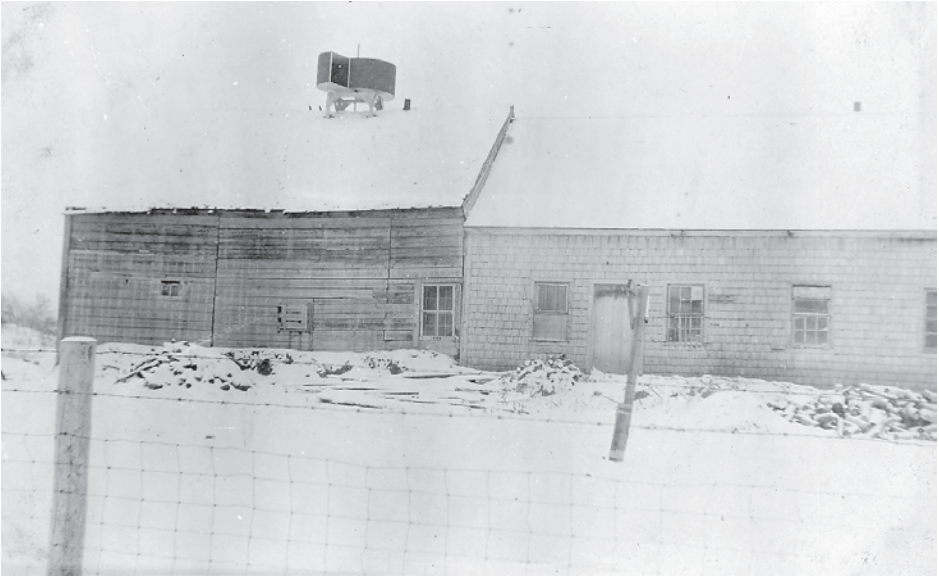
1933. House-barn built by Maria Brandt Plett on Lot 17, presumably as an Anwobner since she only acquired the Feuerstelle in 1883. 912 In 1965 it was the oldest dwelling in Steinbach. Note the windmill device mounted on top of the barn to generate electricity for the owner's use. The building was demolished in 1989 to make way for a new MCC building. Photo - Pres., No. 10, Part One, page 73.
