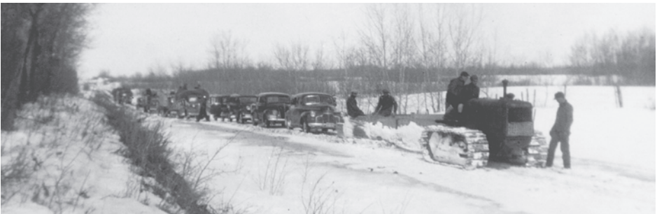
Below: In spring before the frost came out, the lumber camp broke up. On the last day, a caravan of automobiles and trucks wound its way along the rough private logging road built by the Plett lumber company, following the TD35 which dragged the road to make it passable. Photo - Gertrude Friesen Plett, spring 1942, at the intersection on the Highway north of Roblin.
