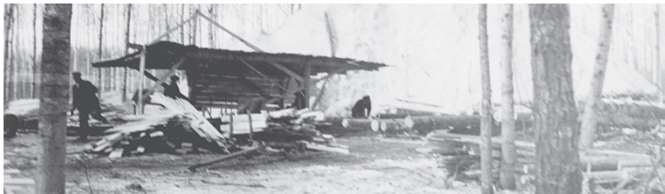
Plett & Co. sawmill at Vassar, 1934, before the steam engine shelter was built. Heinrich E. Plett (left) stepping over the drive belt.
