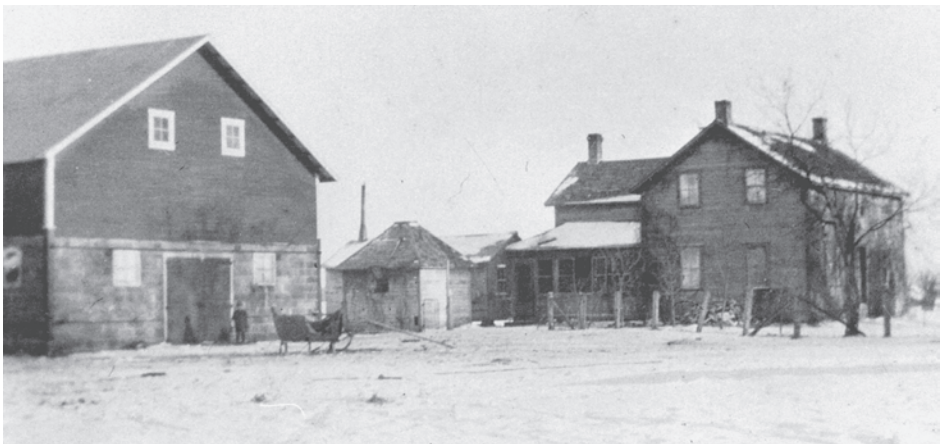
Peter L. Plett yard, SW 35-7-6E, in Blumenhof, Manitoba as it appeared ca. 1930. View to the northeast. It was one of the few barns in the area with the stone mortared walls for the ground floor. Photo courtesy of Sid Barkman.
