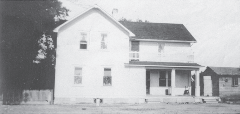
David L. Plett house built in 1920, view to the west.
