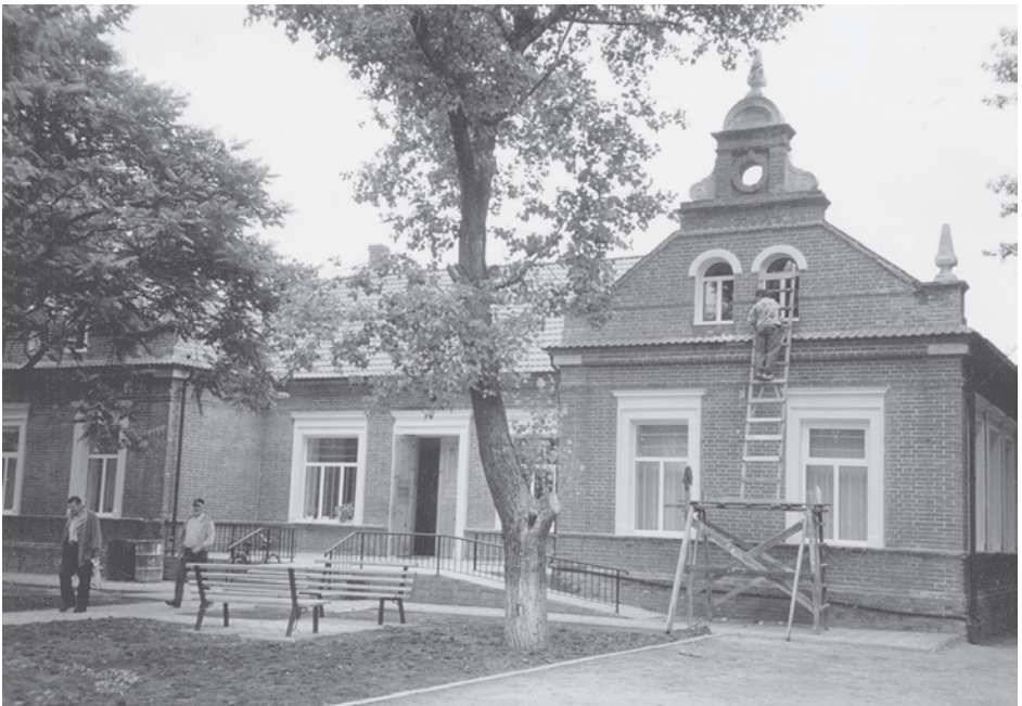
The Girl's School in Halbstadt, built in 1909. In 2000 the building was remodelled and opened as a "Mennonite Centre" to serve as a cultural centre and to provide assistance and education to the local residents. Photo June 2003. See Diese Steine, page 244/Pres., No. 18, page 64.
