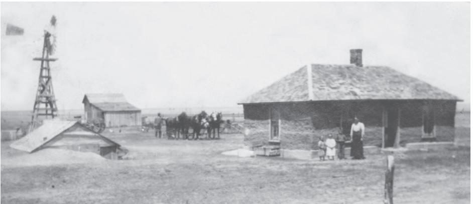
Jakob N. Koop home in Satanta, Kansas, in about 1916. The house is built of adobe. Vegetable cellar to the left. Helena Doerksen Koop in front of the house with her three children. Jakob N. Koop with team of horses in the rear. Photo - Pres., No. 16, page 93.
