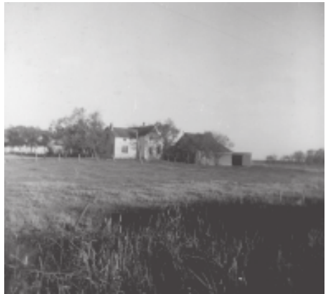
4. Big old house in 16-7-6E. This type was one of the earliest non-Mennonite styles introduced into the East Reserve during the 1890's. Foundation is of fieldstones. There are about 6 of these houses north-west of Steinbach; some built by Clearsprings settlers, others by Mennonites.
