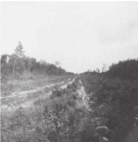
3. Difficulties of road building on the north side of 6-5-6E. Boulders of all sizes are abundant.
