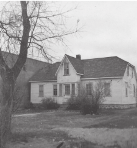
3. House of semi-Mennonite-Russian design on Steinbach's Main Street. The wide front and the bevelled gable ends were particularly characteristic of Mennonite institutions in Russia. Steinbach's first private school had a similar design. This is the only house of this style now left. It dates from about 1900 – note stone and mortar foundation.
