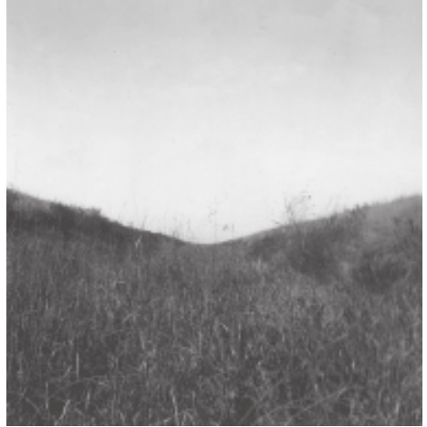
2. Bottom of Manning Canal in 26-7-5E, 1/4 mile from where it begins. The design of the narrow 15-20' ditch, with its steep banks is considered outmoded today because the capacity of the ditch is greatly reduced when filled with snow, and it is therefore liable to overflow in spring.
