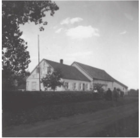
2. "Classic" Mennonite house and barn, built at the turn of the century in Neuborst. Note: shutters, barn door, and the barn windows. Pitch of roof is not very steep because wooden shingles were used. Note flower garden and orchard in front yard. Pediments above the windows are the one embellishment.
