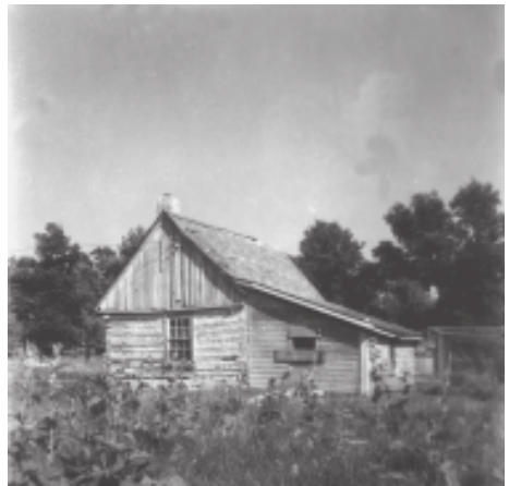
4. Herdman’s house in Bergfeld; built in 1885. Located on outskirts of village. Note that the log walls slant inwards toward the bottom to keep rain from washing away the clay. House is now used for poultry.
