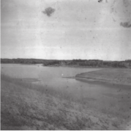
1. Spillway at Morden Dam; and Lake Minnewasta. Dam-height 65'; length 950'. Spillway-width 120'. Depth of reservoir 50'. Reservoir area 143 acres.
