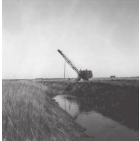
4. Ditch being cleaned – 1 1/2 miles north of New Bothwell. Dirt is dumped on farmer's land to form a levee. A road is on the spoil bank at the left.
