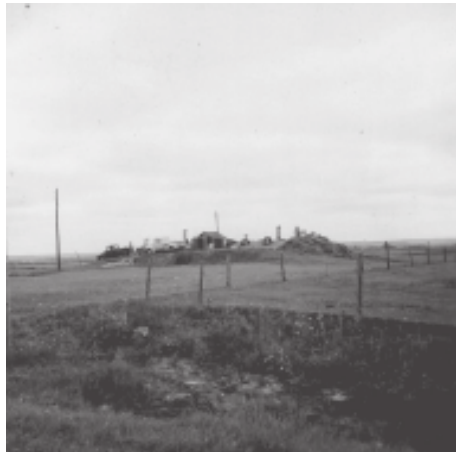
3. Potato cellar just west of Blumenfeld. There are a few of these in the West Reserve-most of them south of Winkler.
