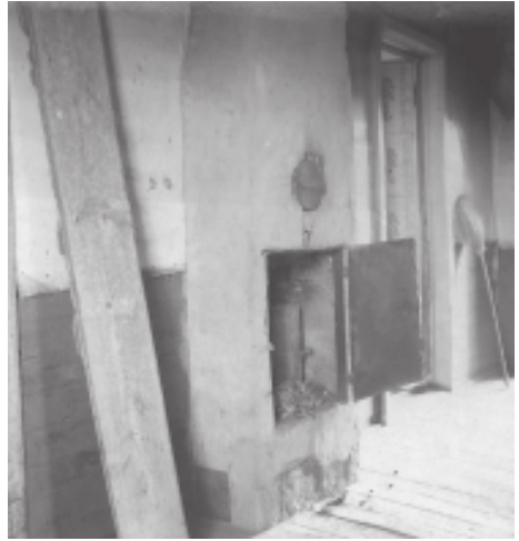
2. Front of the old Mennonite stove. This stove was actually built in the 1920's, but it is the same design as the stoves built in the 1870's and 1880's. The stove was fired through the door shown with straw, or dried and pressed manure, or wood when available.
