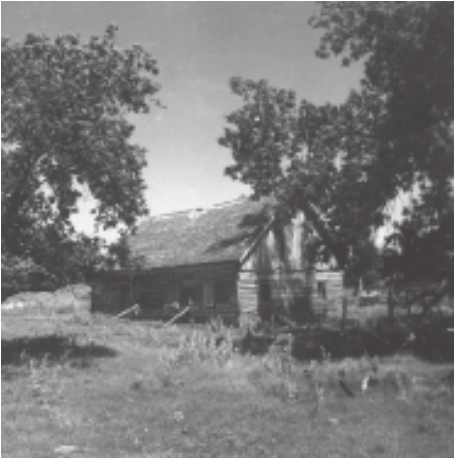
1. Oldest house in Blumenfeld – built in either 1877 or 1878. Dove tailed corners; windows are small and square. Barn has long since been demolished, but the house was lived in until 1945.
