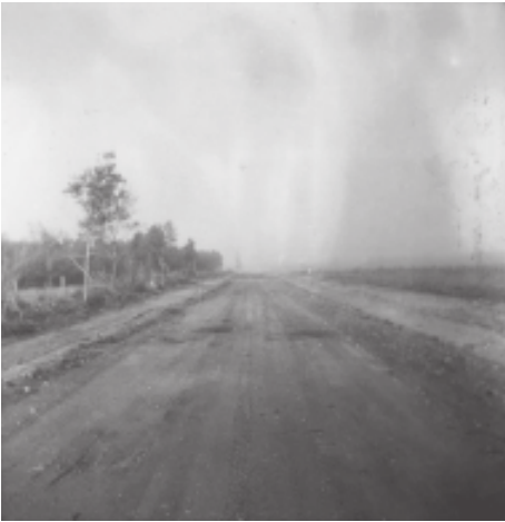
1. This road, on the north side of 20-6-6E on Pelan Stony soil, was quite passable after a heavy rain even though it is not gravelled. Has a firm road base formed of the gravelly soil. On this same morning roads to the north of Steinbach on the Blackearth soils were impassable. Bush on the left; recently cleared land on right.
