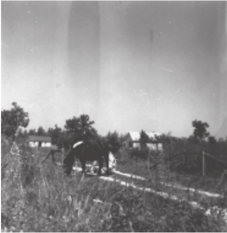
1. A new farm being cut out of the bush in 29-6-6E. Farmer has a few cows and a small acreage of sugar beets. Horse power is still being used.
