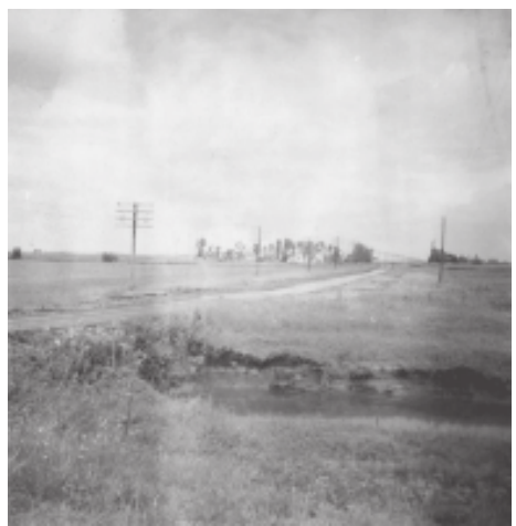
4. Double dyke in 33-3-1W. Asphalt on road in order to allow vehicles to cross even when there is water between the dykes. This only happens in spring when the ditch in the foreground can't hold all the run off.
