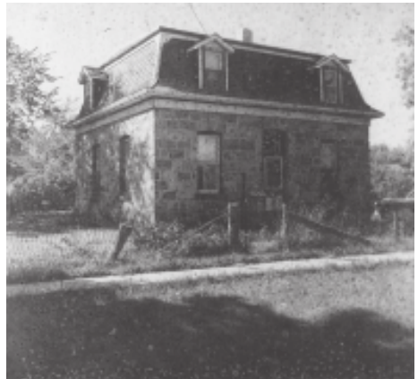
4. Stone house in Morden; built at the turn of the century. Blocks are roughly squared glacial erratics. These buildings are only found on the Reserve at Morden. A number of these buildings have been erected in other villages to the west. No Mennonite ever built one, although in the late 1890's one or two Mennonites who farmed in the Morden area built brick homes.
