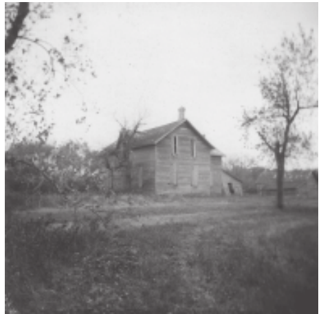
3. Abandoned, 60 year old Ontario settler's home; south of Darlingford. These rather austere frame farm houses, which antedate the ginger bread period of the early 1900's, were characteristic of the Ontario settlers. Mennonites at that time were still building their houses and barns together.
