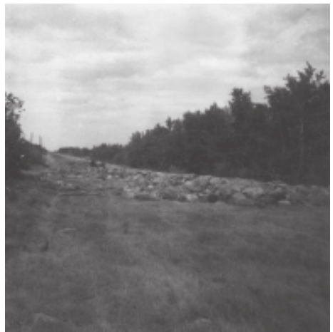
4. Raising the grade against spring flooding in 24-5-6E. Shows why so much of the land is used for pasture in the southern part of the East Reserve – the rocks were removed from just below the surface of the smooth sod. In this area one Lake Agassiz beach follows another producing these terrain conditions.
