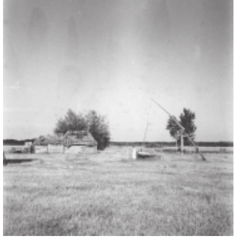
2. Ukrainian house in 12-6-6E; built in 1902. Only house left in the East Reserve with a thatched roof. Well sweep is still typical of Ukrainian farms in the Reserve.
