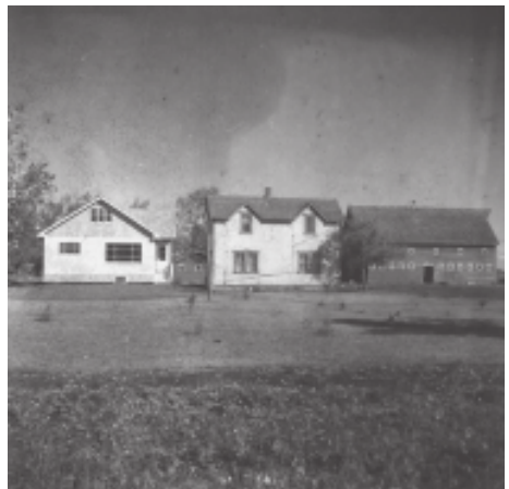
4. Contrast in farm houses in 19-3-2W. Old house built about 1910, is typical of the houses built at that time, though not many people had enough money to build them as large as this. Squat barn is also typical of the time. Foundations are of mortared stone. New 1 1/2 storey house is being built in 1955; it has all the conveniences; also a bright colour scheme.
