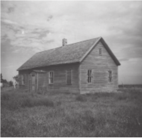
1. Abandoned Mennonite private school in the village of Rudnerweide, west of Altona. Teacher lived on one side, the classroom was on the other. Contains the stove shown in the following photographs.
