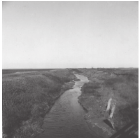
4. Manning Canal in Tache Municipality (22-8-4E). Spoil banks on both sides are well above the countryside. The canal here is 15-20' deep.
