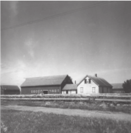
3. Sommerfeld; showing the long axis of the house perpendicular to the land axis of the barn. Every house in Sommerfeld is oriented this way – probably for hygienic reasons. Shutters are a conspicuous feature of the Mennonite house. The connecting passage between the house and barn is well shown. Note the size of the barn door now that bay is hoisted into the loft via the gable.
