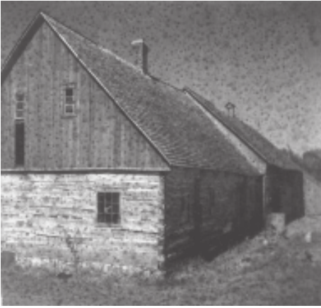
1. Log House, 3 1/2 miles west of Chortitz. Built in 1876, in village of Waldheim 1/2 mile to the east, but moved here the next year when some of the villagers decided to move on their quarter sections. Big logs were hauled from Pembina Mountain, field stones for foundations obtained locally. Beautiful dove-tailed construction, especially for the Mennonites, who had only been here for one year and had no previous experience in building log houses. There were no Red River style houses in the West Reserve. Note the steep pitch for straw roofs.
