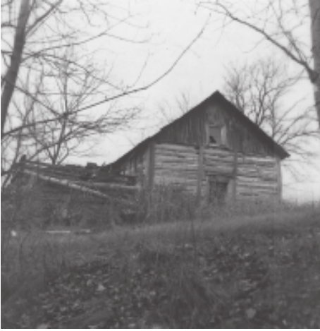
1. Metis house on Seine River, east of Ste. Anne, 16'x16' with saddle and lap corners. Inside was plastered, using willows for lathes. Mennonites built larger homes than this and therefore used the Red River style.
