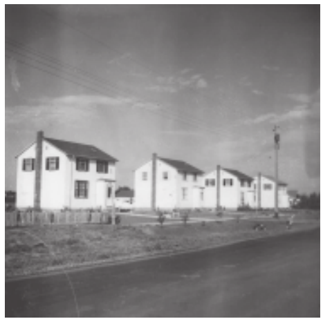
4. On one hand Gretna is a museum piece among West Reserve towns, on the other hand it is just as unique in having a small scale housing development. These houses were put up by the Pipe Line Company for their Gretna Pumping Station employees.
