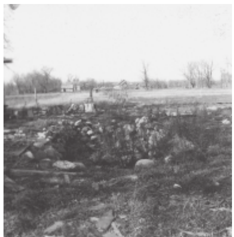
4. Bergfeld: cellar of a dismantled house. The cellar is three feet deep and lined with field stones.
