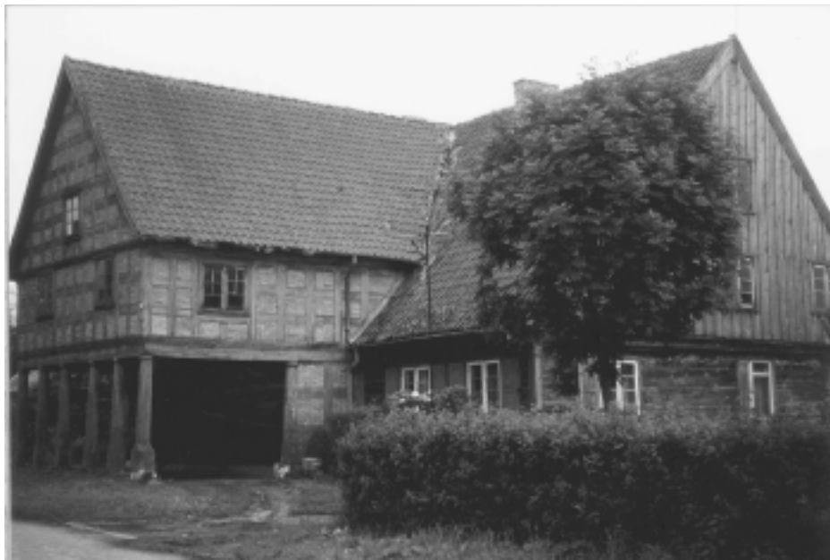
A Mennonite Vorlaubhaus (arcaded house) in Lubieszew, formerly Ladekopp, West Prussia/Poland, possibly dating from the 18th century. A beautiful example of this type of building, many of which are still in existence. Photo by Ron and Wendy Dueck, Kleefeld, Manitoba, 1996. Photo courtesy of Pres., Part Two, page 59.
