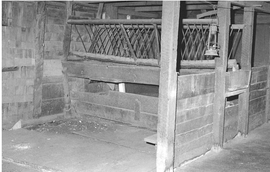
Double crib and trough for six horses in the Rempel-Ens housebarn. Photo by Henry G. Ens.
