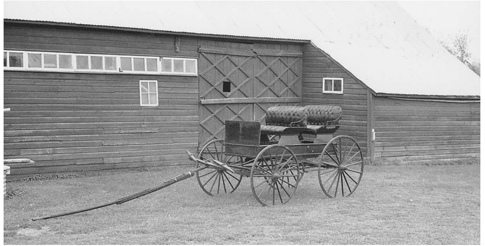
Closeup showing the main entrance into the Scheune (hay mow) where equipment such as buggies and wagons were stored and feed for the livestock was stockpiled for winter. Note the row of high small windows, typical in earlier Mennonite barns, and the detailed cross bracing of the double barn door. The original part of the barn dates to ca. 1880. The buggy was purchased by Abram Rempel in 1915. Photo by Henry G. Ens.
