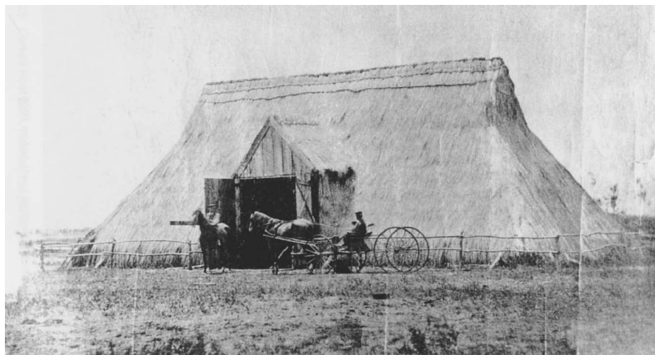
A more elaborate Sarais, built circa 1875, by an Old Colonier in the West Reserve, Manitoba. Photo courtesy of Frieda Klippenstein, Neubergthal...Landscape History (Parks Canada, Winnipeg, 1997) , Illustration 22/Preservings, No. 16, page 137.
