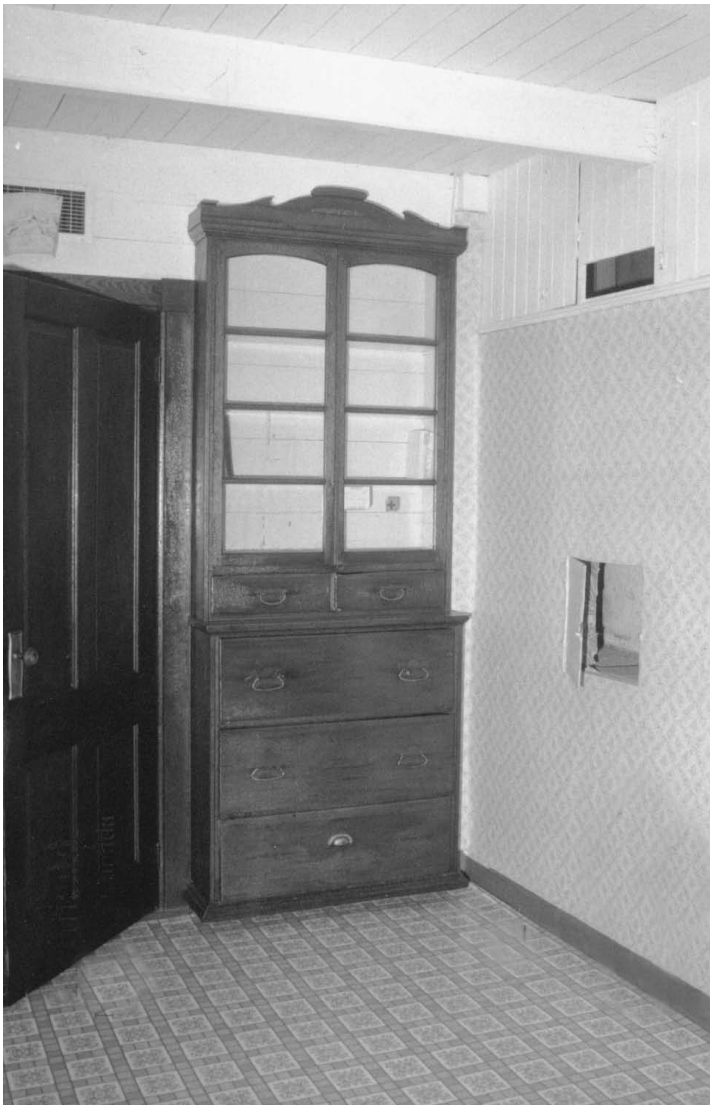
A built-in china cabinet ("Miraschaup") in the Atjschtove. Note the door to the internal central hearth, on the right. View to the west. This housebarn features a second built-in china cabinet with drawers in the Grootte Schtove. Photo by Henry G. Ens.
