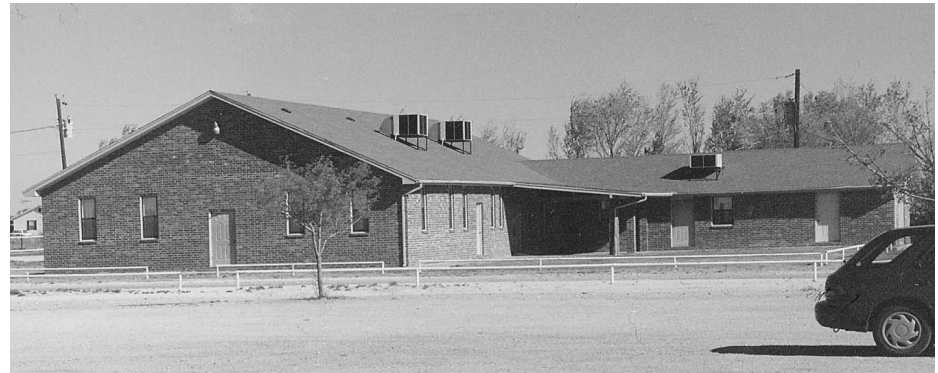
1996 The Old Colony Mennonite Church in the "Airport subdivision" just south of Seminole, Texas. The building has electric lights and air conditioning. Photo by Tony Enns, Winnipeg, MCC Kanadier Committee, and courtesy of Henry Unger, Box 181, Crystal City, Man., R0K 0N0.
