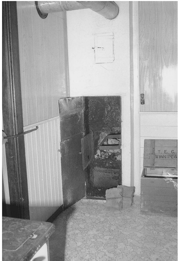
The kitchen door of the Tiajel-owen (the central brick heater), a feature of traditional Mennonite housebarns, is still intact. The internal brick oven was built literally in the centre of the house, so that most rooms were adjacent to it, thus minimizing the need for ducting. The central brick oven and chimney were built in such a way as to create a simple Riatjakoma (meat-smoking chamber) on the second floor, used to smoke hams and sausage. Photo by Henry G. Ens.
