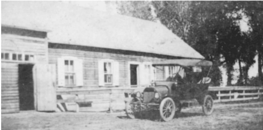
This Wirtschaft belonged to Jakob Enns in Rosenort, W. R., Manitoba. The buildings were built completely new in 1917 when the original buildings were totally destroyed by fire. Photo and caption courtesy of 75 Jahre Mennoniten in Mexiko (Cuauhtemoc, 1997), page 16.
