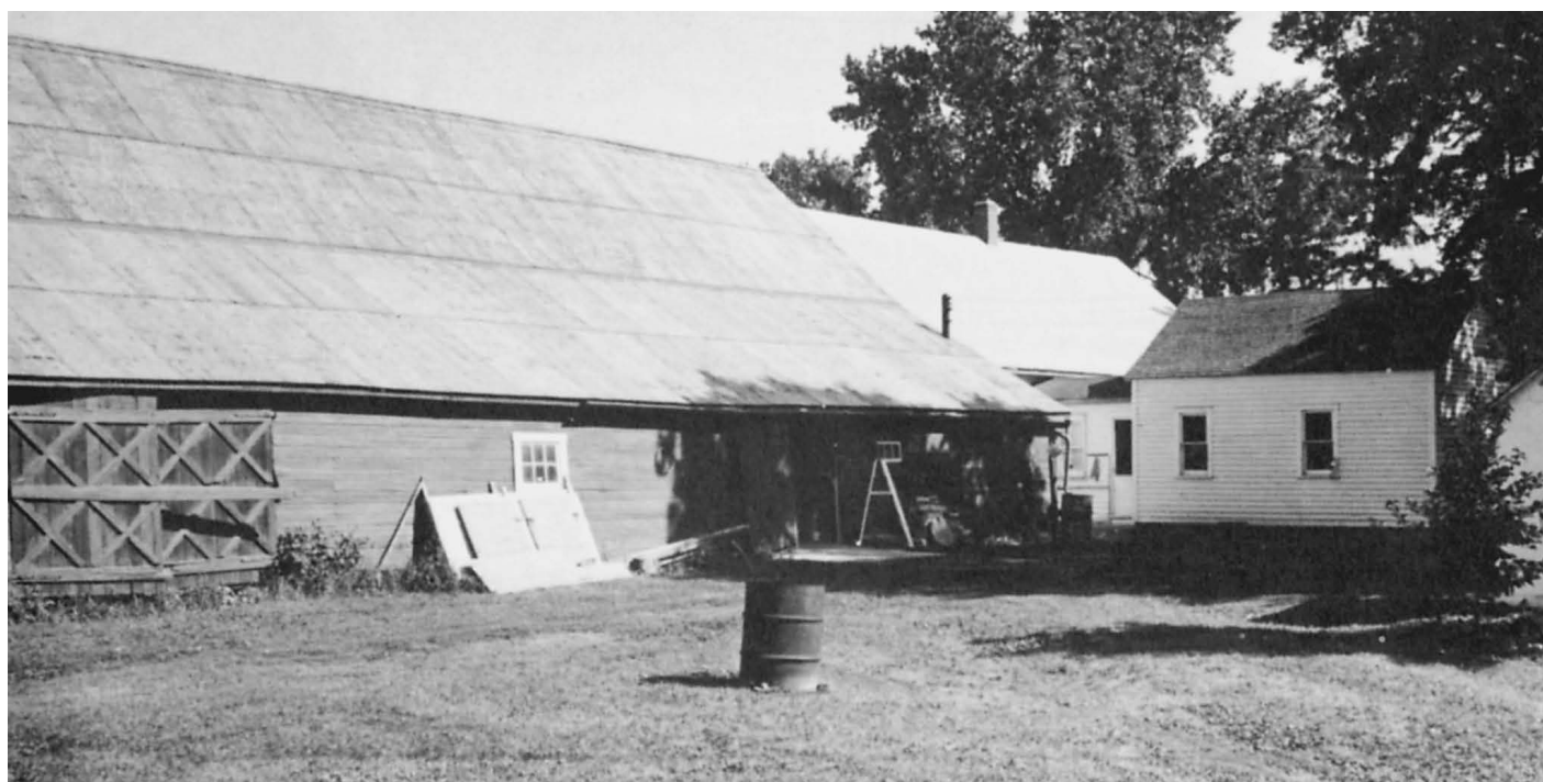
The Rempel/Ens housebarn, view from the northwest, presenting the linkage between the house, the barn, and the summer kitchen to the right. The "Gang" or gangway between the house and summer kitchen was unique. The feature was commonly used to connect house and barn in prairie housebarns by the turn-of-the-century, but the summer kitchen was usually free standing. These innovations reflect adaptation to local building materials and styles. Photo by Werner Ens, courtesy of Peter Zacharias, Reinland (Altona, 1976), page 95. A detailed floor plan of the house and barn, as well as an aerial photograph showing the outline of the structure, have been published by Zacharias, Reinland, pages 98-99.
