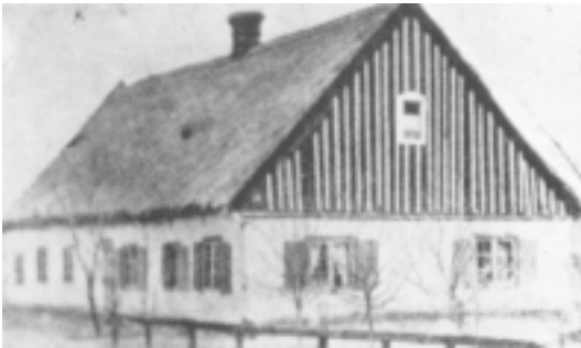
The old school building in the village of Margenau, Molotschna, which was used until 1850. Margenau had a significant KG community and for some years Cornelius Friesen (1810-92) was the school teacher there.
