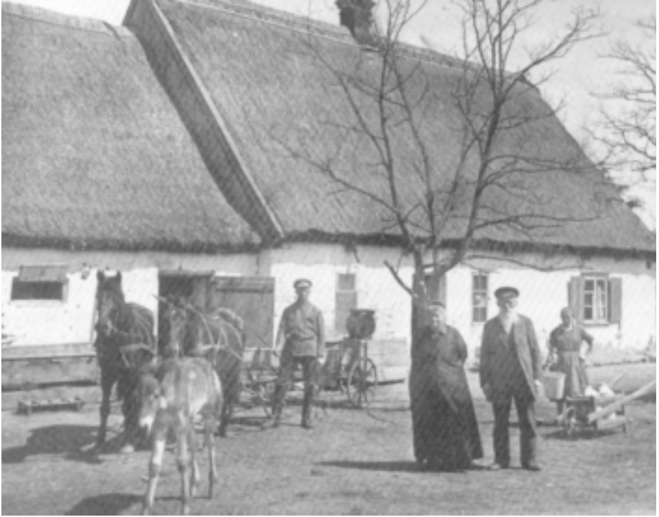
An old housebarn in Blumenort, Molotschna, built of bricks with thatched roof and attached barn as in Prussia. The house is reminiscent of the traditional longhouse or housebarn once common in the Lower Saxon /Friesland area from which many of the Mennonites had originated in medieval times. Blumenort was the home of a number of KG families in the early years, including the wealthy Johann Warkentin (1760-1825), who chose the name of the village, his son-in-law Heinrich Friesen (1786-1842), Peter Brandt (1770-1819), and Gerhard Goossen (b. 1778).
