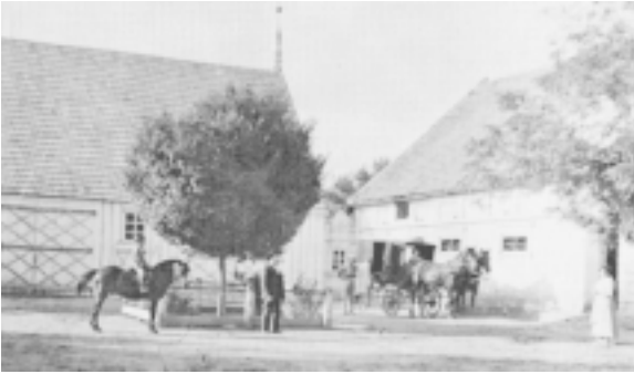
A new style farmstead in Obrloff, Molotschna. The family is getting ready to go visiting in their "Vordeckwagon", an enclosed carriage still commonly used among Mennonites in Mexico and Bolivia. Six KG-associated families have been identified in Obrloff in the 1835 census. Photo courtesy of Gerlach, Bildband zur Geschichte der Mennoniten , page 75.
