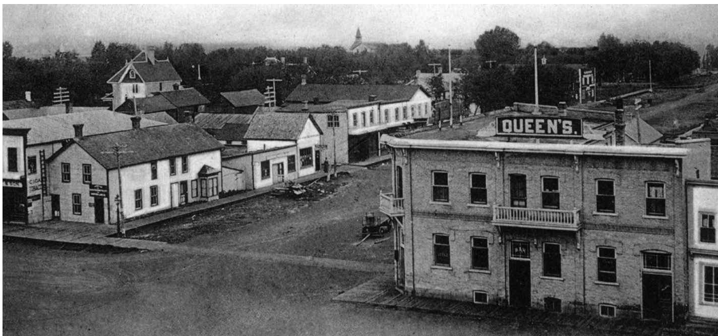
A view of Gretna taken from one of its two grain elevators, which impressed Alekseev for their efficient operation.
