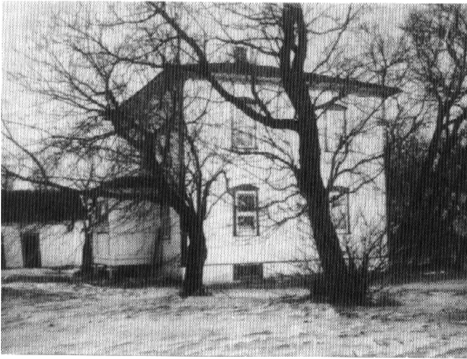
New house built by Cornelius C. F. Toews in 1916 which burned down in 1991. Photo courtesy of Elma Peters Plett.
